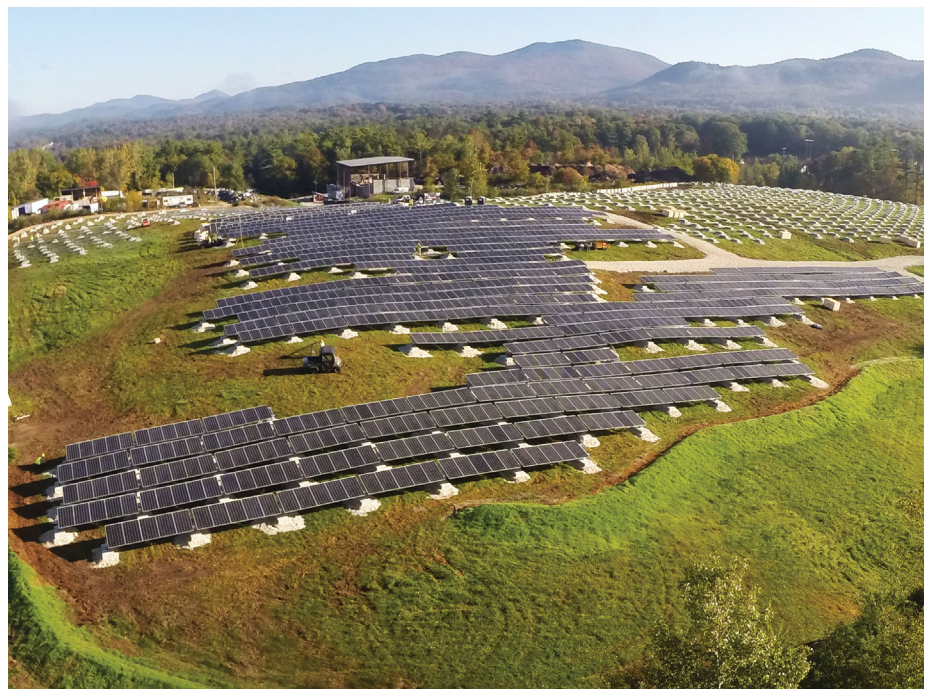
Green Mountain Power built the 2 MW Stafford Hill solar farm on a closed landfill. Vermont's burgeoning solar sector is producing innovative tax models. Photo courtesy of Green Mountain Power
