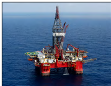
Associated Press The Centenario deep-water drilling platform stands off the coast of Veracruz, Mexico, Nov. 22, 2013.
